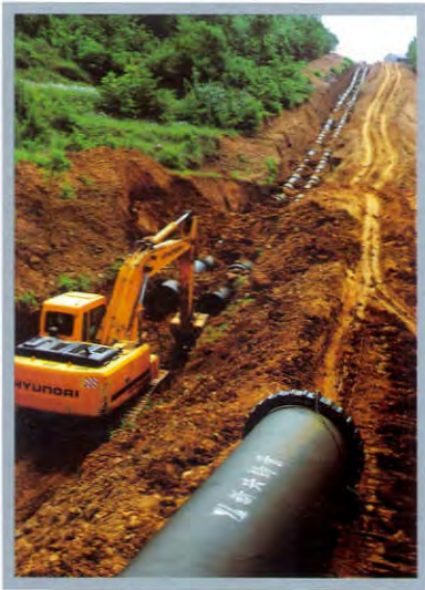
郑州平顶山电厂项目新兴铸管开创了在地势错综复杂的情况下铺设球管的先河 Pingdingshan Power Plant Project in Zhengzhou, Xinxing Pipes has pioneered the way of laying ductile iron pipes in the case of complex terrain
