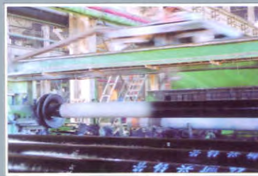
沥青涂覆 Bituminous coating
